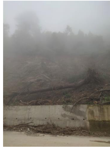
(h) Semali Katal landslide
