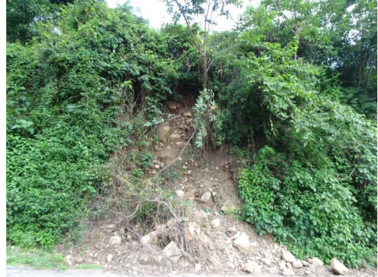
(f) Dhaulangi landslide
