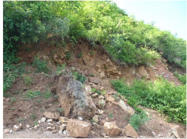
(b) Jhaki dagar 2 landslide
